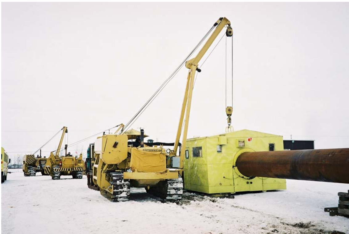
Fig. 1: System configuration: Crane, welding tent, thermobox, truck – real-life conditions/
