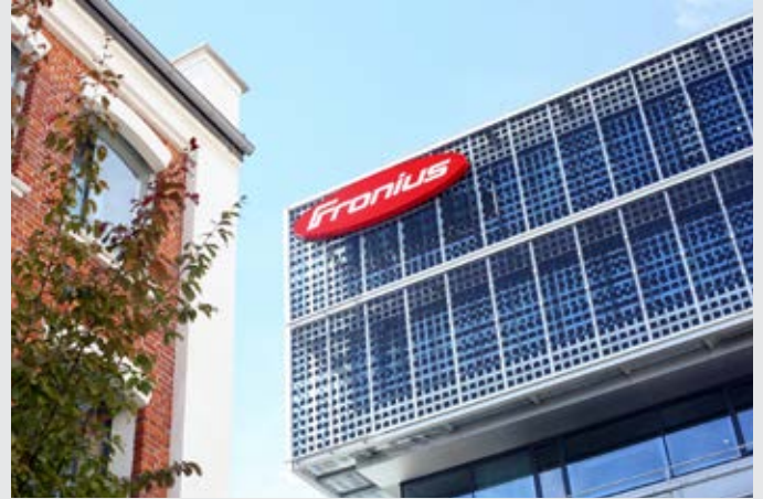
/ The building's heating and cooling requirements are covered by a combination of geothermal energy and solar power.
