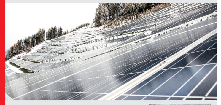
/ With an output of 3.15 MWp, the PV power plant in Flachau is currently Austria's largest field installation. The system is south-facing and lies at 1,200 metres above sea level in a meadow grazed by sheep.
