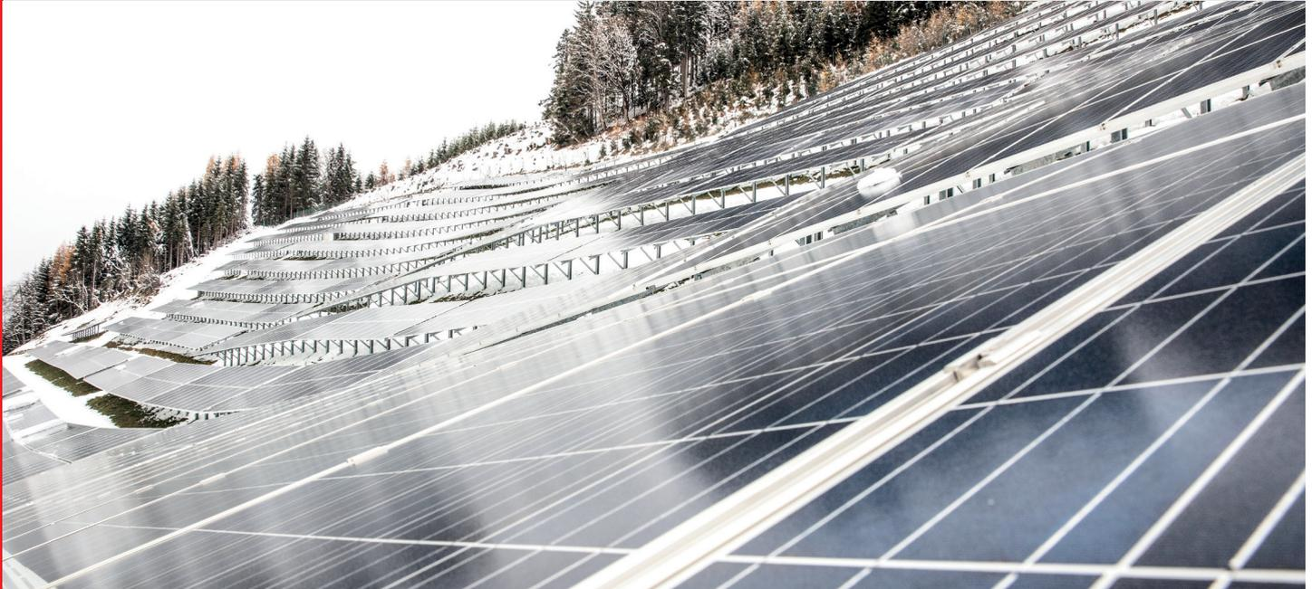
/ With an output of 3.15 MWp, the PV power plant in Flachau is currently Austria's largest field installation. The system is south-facing and lies at 1,200 metres above sea level in a meadow grazed by sheep.
