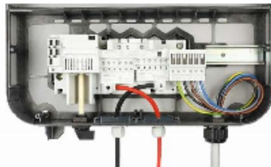
/ The DC connector kit enables the connection of both inputs in the event of MPP currents above 35 A and a cable cross section of more than 16 mm<sup>2</sup>, for example when using a DC Box. A cross section of 6 mm<sup>2</sup> - 25 mm<sup>2</sup> can be connected using the DC connector kit. The terminal is safe to touch. The DC connector kit is particularly suitable for use with the Fronius Symo 10.0 - 20.0 kW and Fronius Eco inverters.
