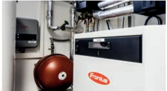
*“Originally a no-go, it now makes perfect sense to heat water with solar energy,”* reports Peter Maul from Hardy Barth GmbH. *“The Fronius Ohmpilot makes it possible. It can be integrated into an existing photovoltaic system and connected to the existing heating element in the boiler.”*
