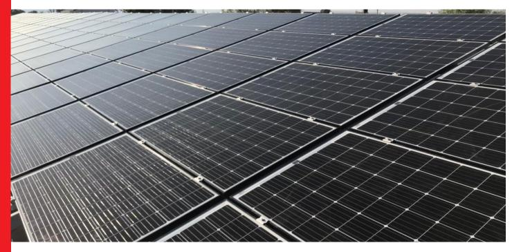
/ One of our most loyals FSP Plus, SMG Global, had the opportunity to develop the third stage of a PV project in the company TEC Engineering. The end customer demanded high quality in all the components that were going to be used, so SMG Global decided to use components and devices with the correct certifications so they could guarantee the works. The system consisted in 504 PV modules of 295 W, 6 Fronius Symo 15.0-3 208 and 2 Fronius Symo 22.7-3 480.
