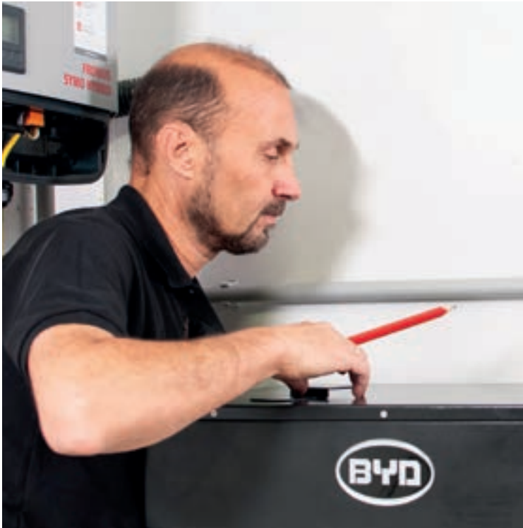
Fronius PV expert Hans Pelzer installing a BYD Battery-Box HV
