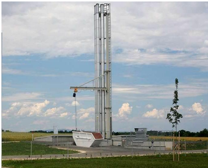
Biomass heating plant in Sattledt covers 80% of the heating requirement
