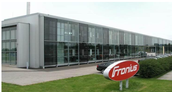
At the Pettenbach site, a climate protection façade has been erected with glass-integrated PV elements.
