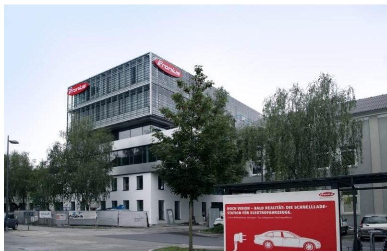
Active Energy Tower (energy-independent renovation in Wels)
