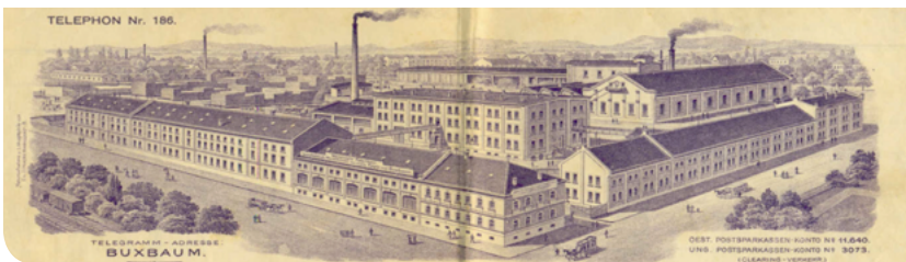
1 / Wels / The historic brick buildings were modernised to make them energy efficient, allowing them to be retained.
